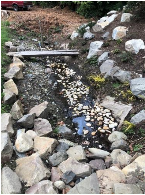
Photo 9. View of the open or daylit section of the Type Ns stream including fresh side slope soils, grading, rock, erosion control fabric, and river rock within the bottom of the channel, looking north. Photo taken 3-17-22.
